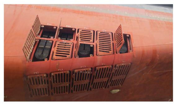
A set of Box Cooler manufactured by Nederlandse Radiateuren Fabriek (NRF) installed in the aft portside sea chest of a vessel.
